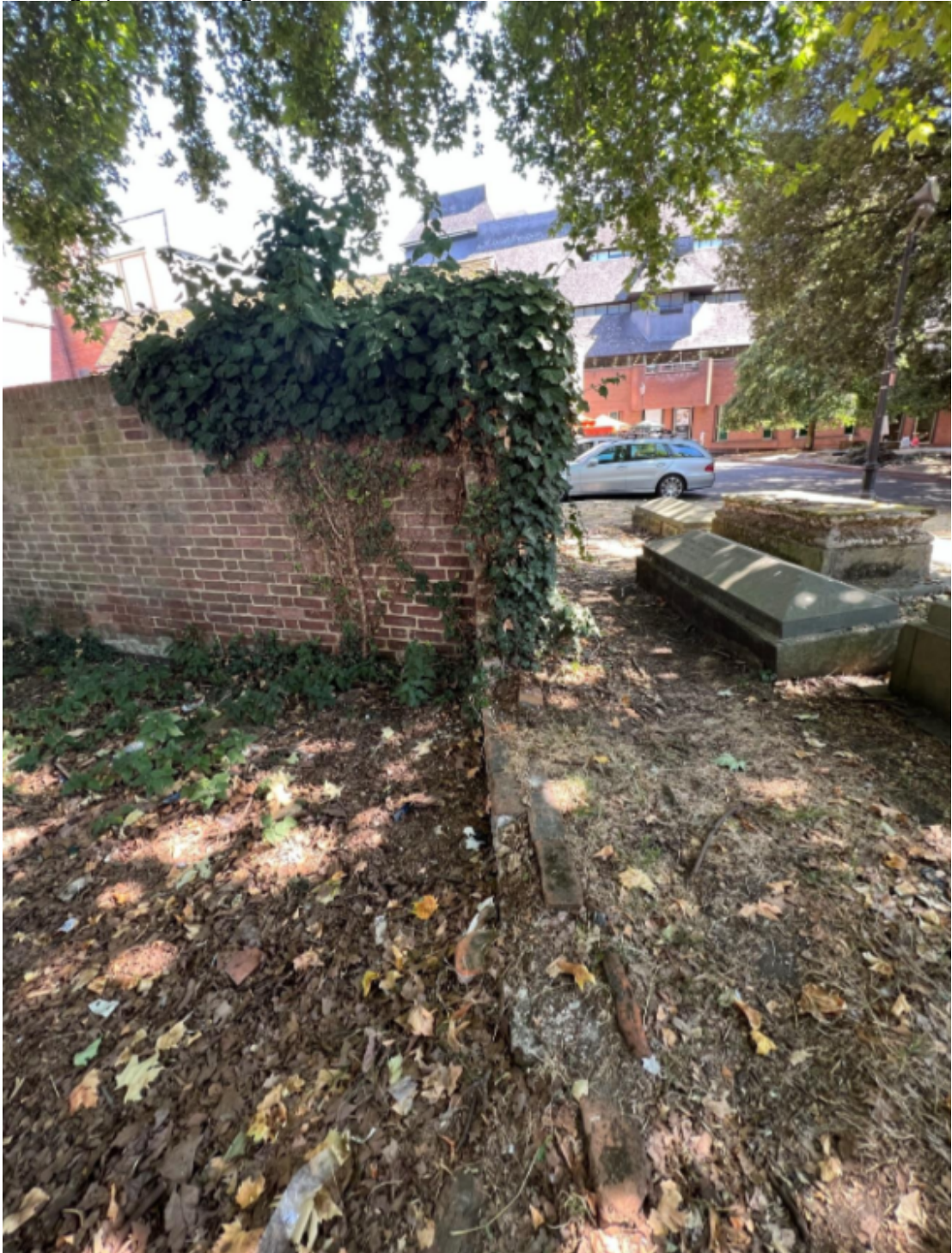
5. Photograph of existing historic wall foundations
