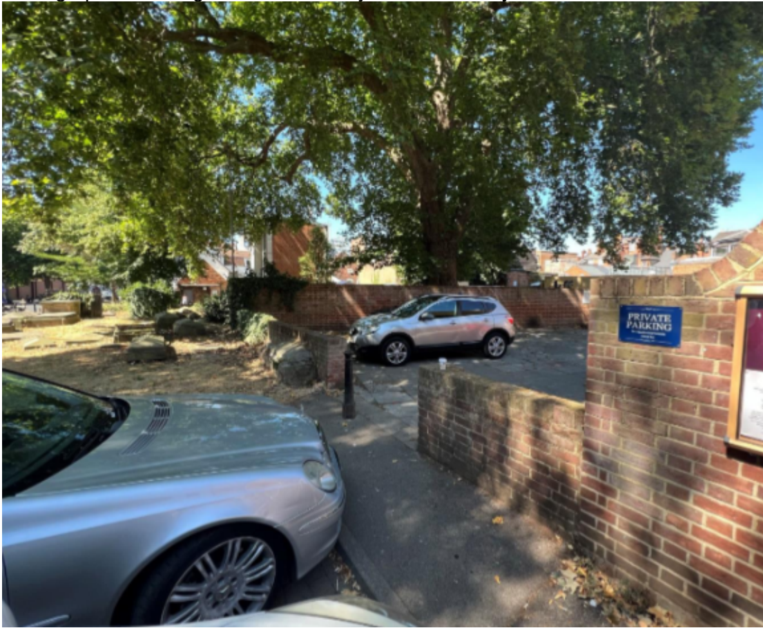
6. Photograph of existing half brick wall adjacent to St Mary's Church House
